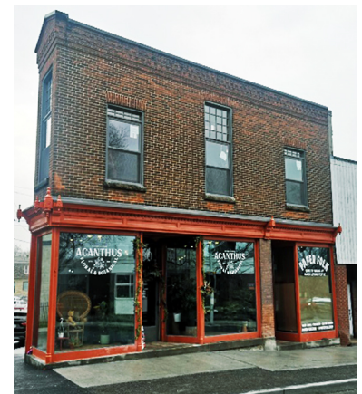
56-60 Mill Street after its restoration in 2022
