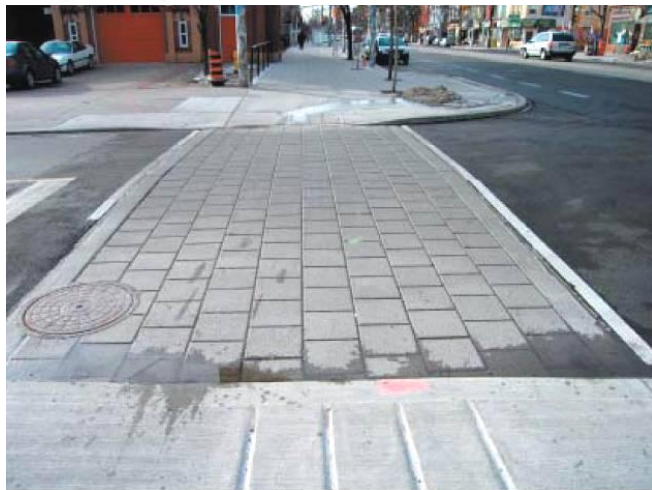
Figure: Crosswalks should be designated for safety, with appropriate surface markings or variation in construction material.
