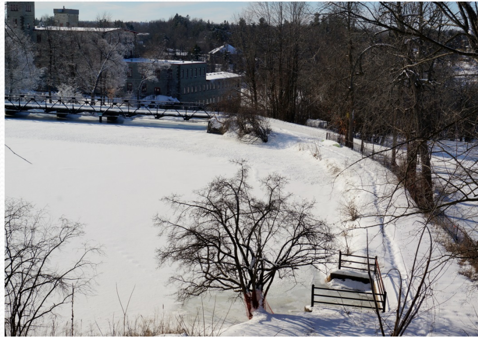
View from OVRT/CPR Trail at Workers' Staircase – Bridge & River Pool
