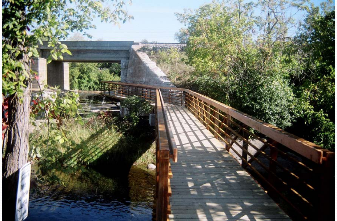
Riverwalk Bridge continuing under Railway Trestle
