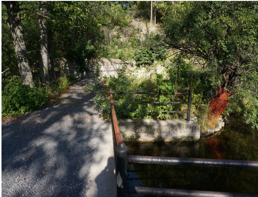
Workers Staircase Rock face & Earthen Dam Track
