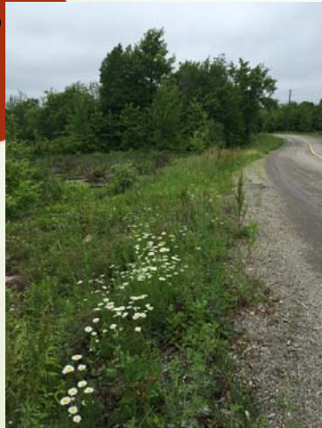
Narrows Lock Road, Unsprayed
