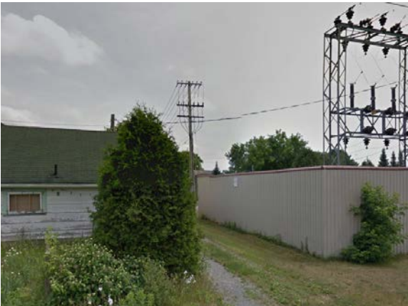
PROXIMITY TO SUBSTATION
