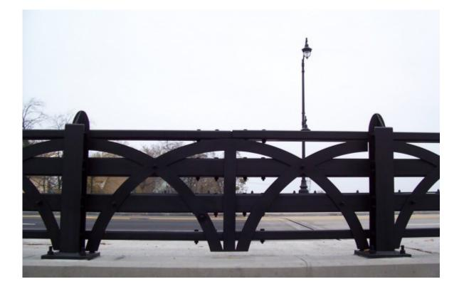
Option 2 - 4-Box steel railing with 'arched' steel panel profile c/w concrete end walls
