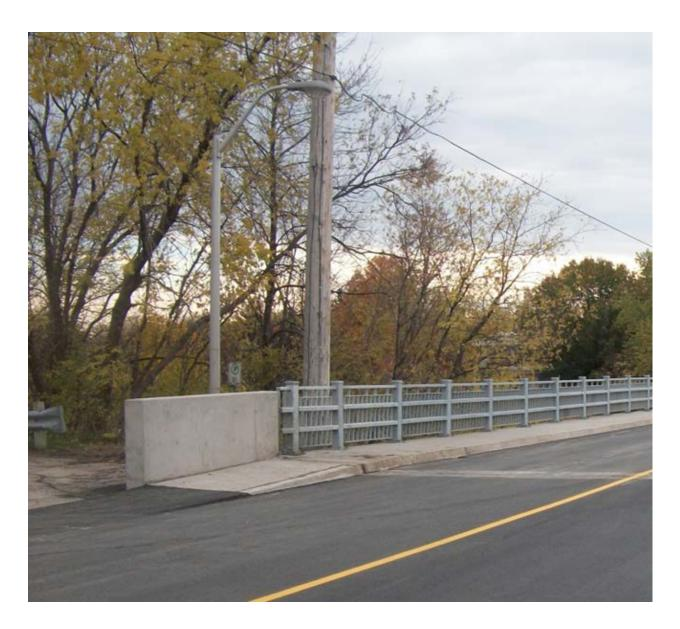
Option 1 - Steel railing c/w concrete end walls
