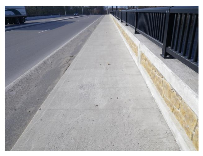
Option 3 - Concrete parapet with decorative finish and steel railing
