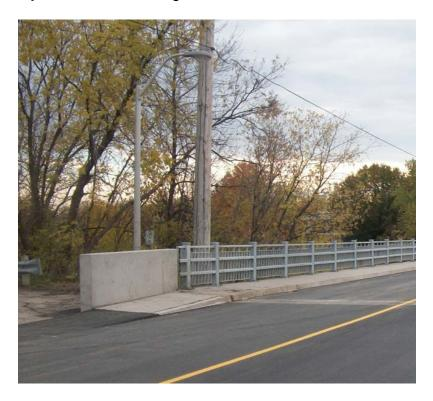
Option 2 - 4-Box steel railing with 'arched' steel panel profile c/w concrete end walls
