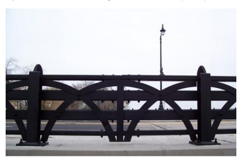
Option 3 - Concrete parapet with decorative finish and steel railing
