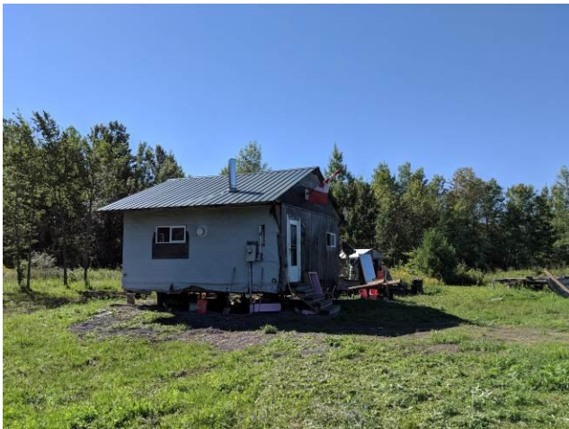
Close-up of Structure
