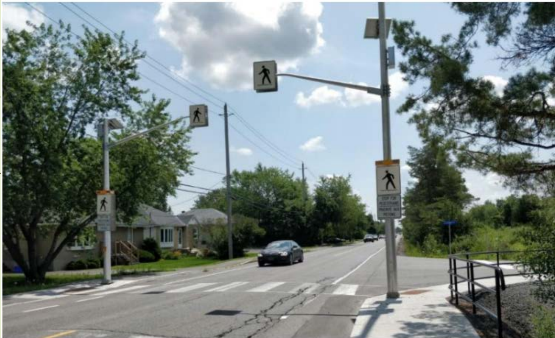
Figure 3 – Image of Type B PXO Located at Blair Road at Appleford Street
